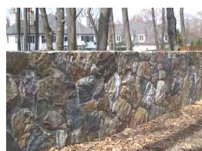
Mortared stone wall
