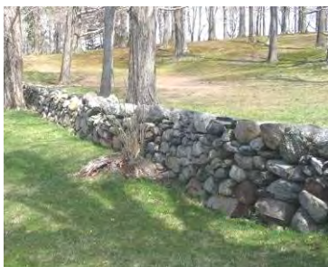
Dry-stack stone wall
