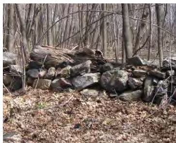
Dry-stack in disrepair
