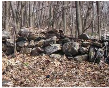
Dry-stack in disrepair
